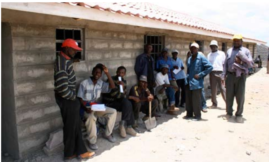
Building Kaputei is a team effort by Jamii Bora's members.
