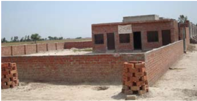
A primary school takes shape at KKB-4
