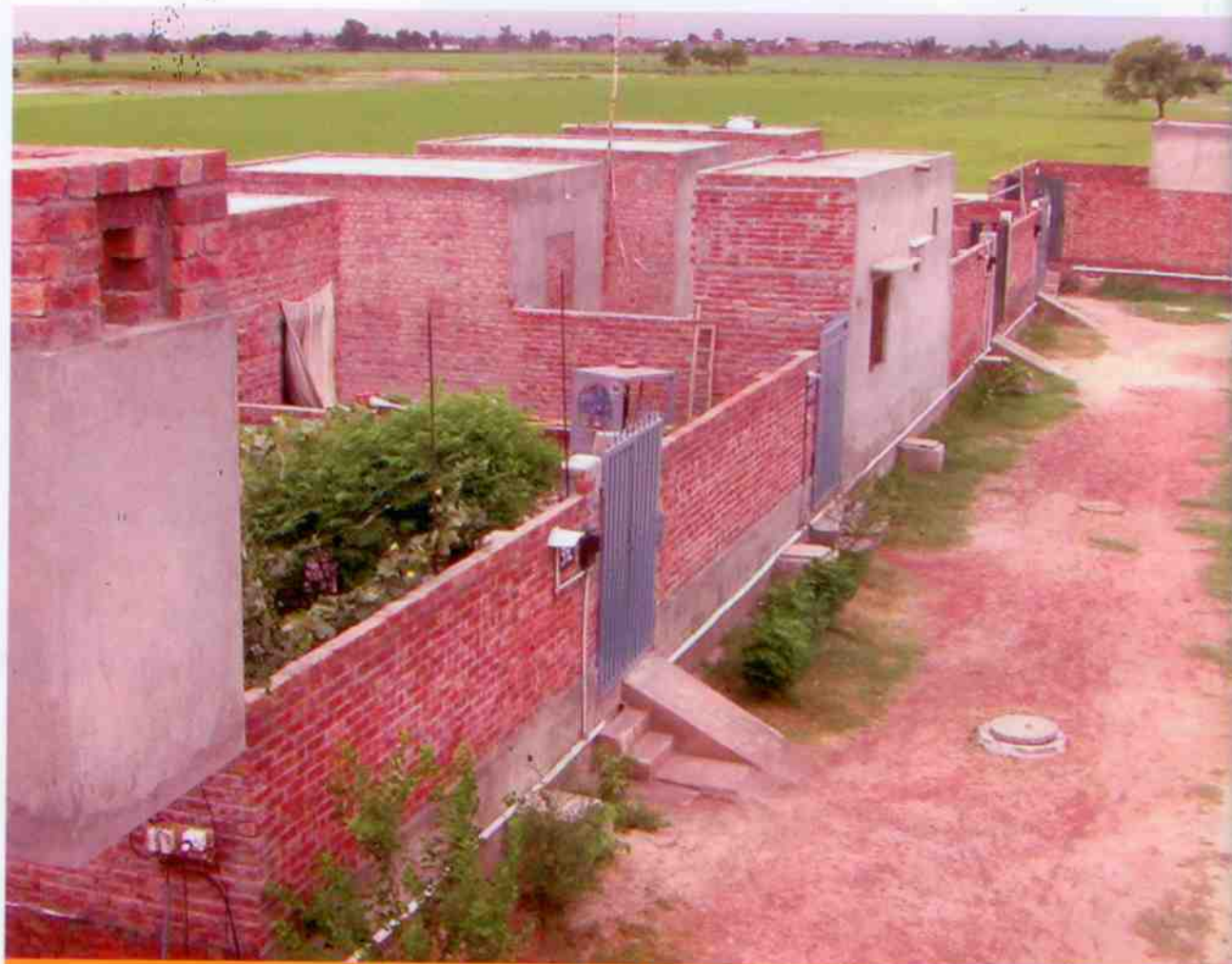
Above and opposite: The Salban housing scheme
